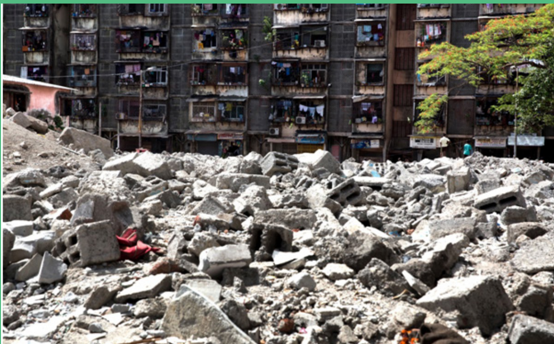
Image 1: Demolition and rehab housing in Mumbai
