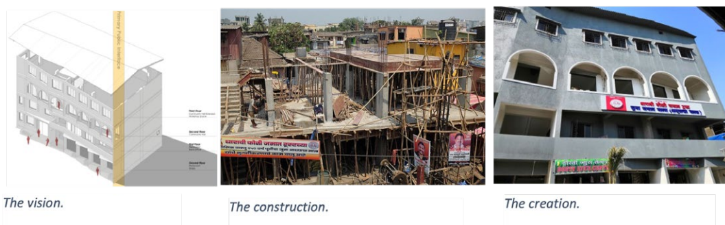
Figure 1: The Construction of the Koli Jamat Community Hall at Koliwada, Dharavi
