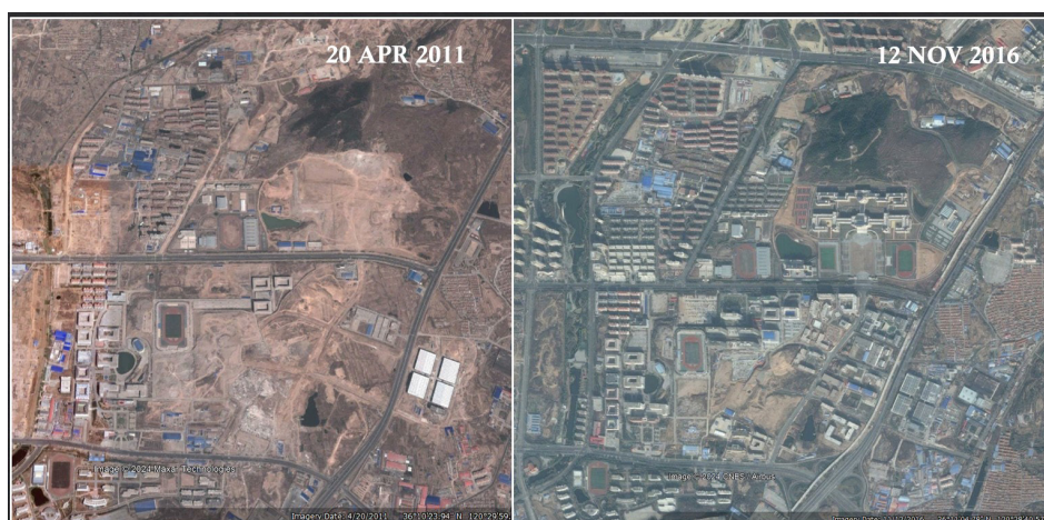
Figure 5: Construction of the NSA (New Complex)
