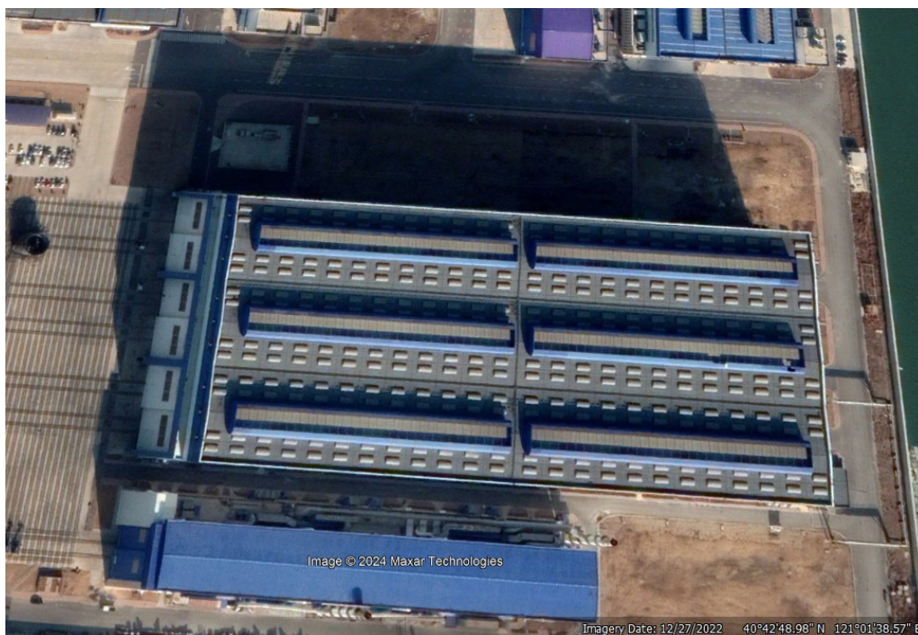
Figure 10: Final Assembly Hall
