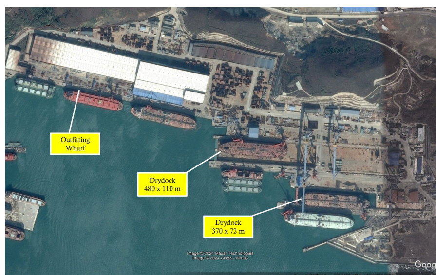
Figure 4: Newly Constructed Outfitting Wharf and Drydocks for Commercial Use
