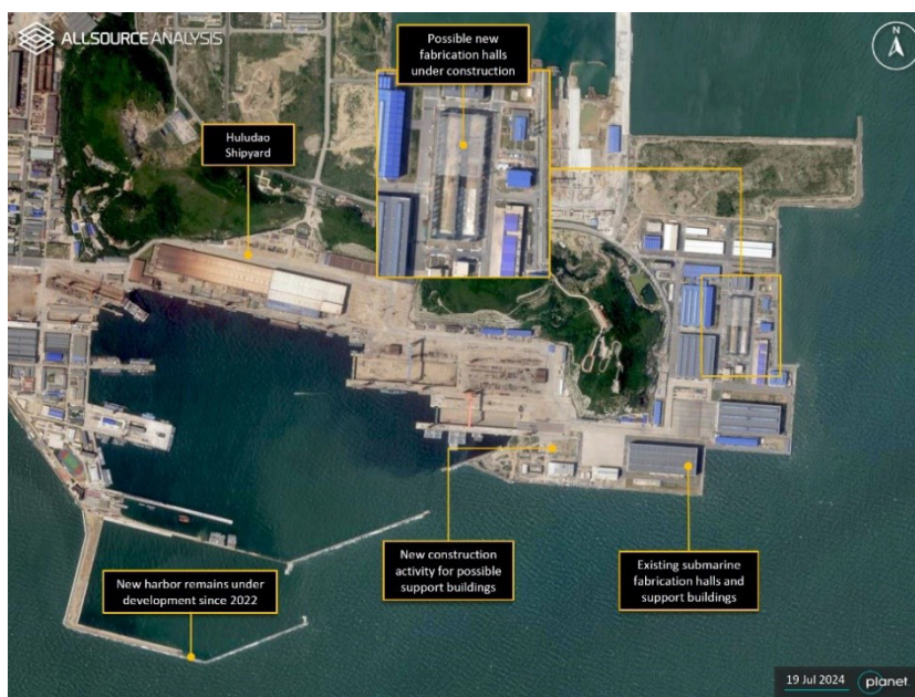
Figure 15: Additional Facilities Under Construction
