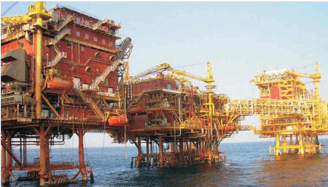
ONGC platform at Bombay High
