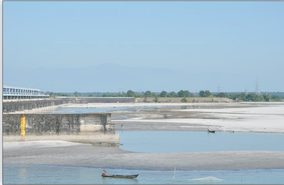
Gazaldoba Barrage on the Teesta River. The water on the other side of the gates has been channeled into irrigation canals.
